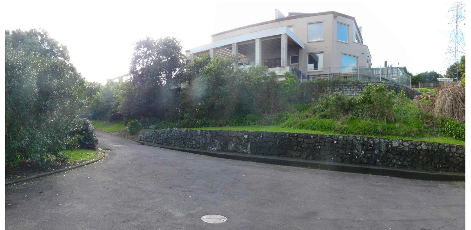
View on site, looking towards access road
